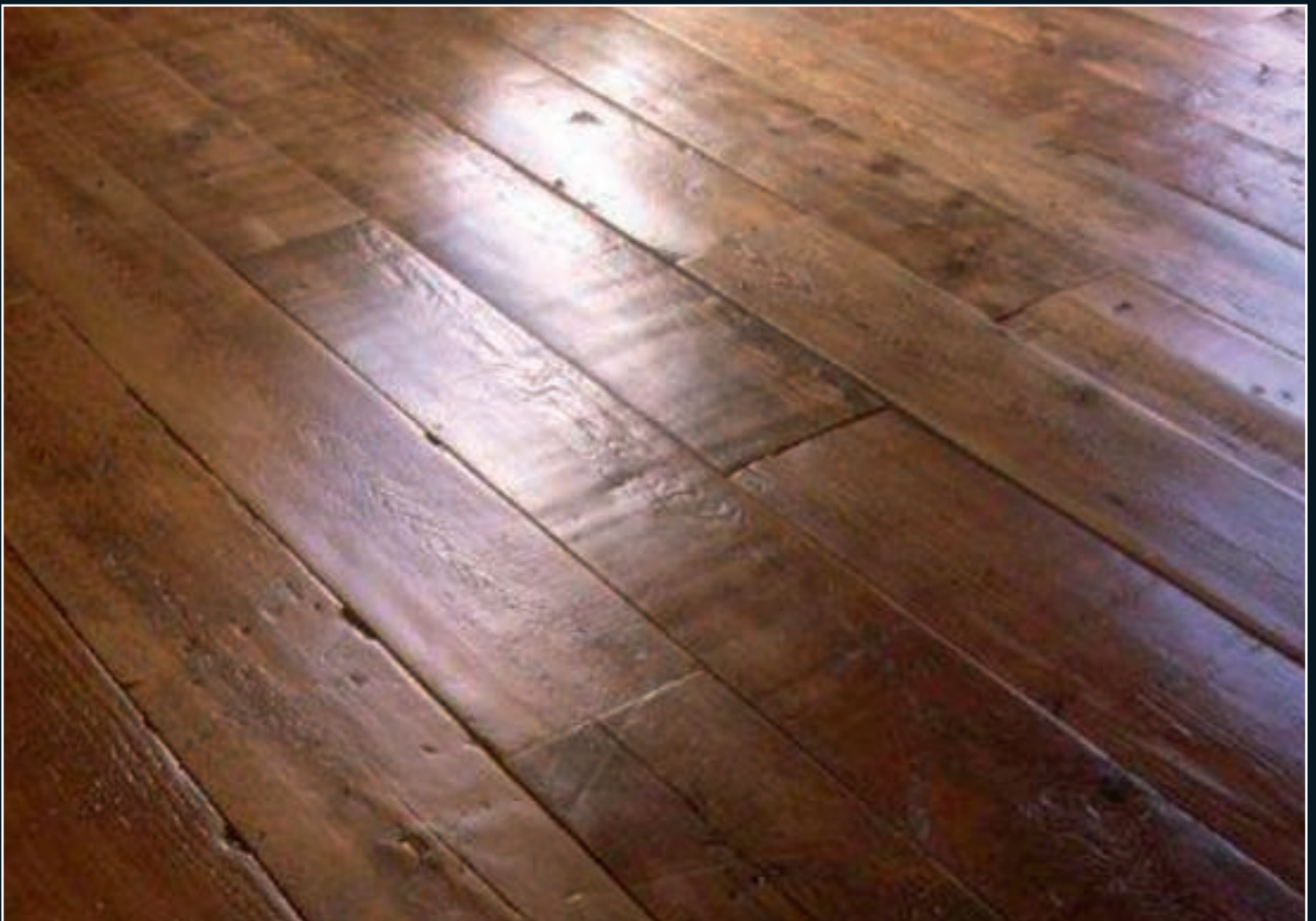
Chester Sq Texture. 1780's Grade 1 listed property in Hampstead. VWW Oak Tint 3. Full waxed finish.
