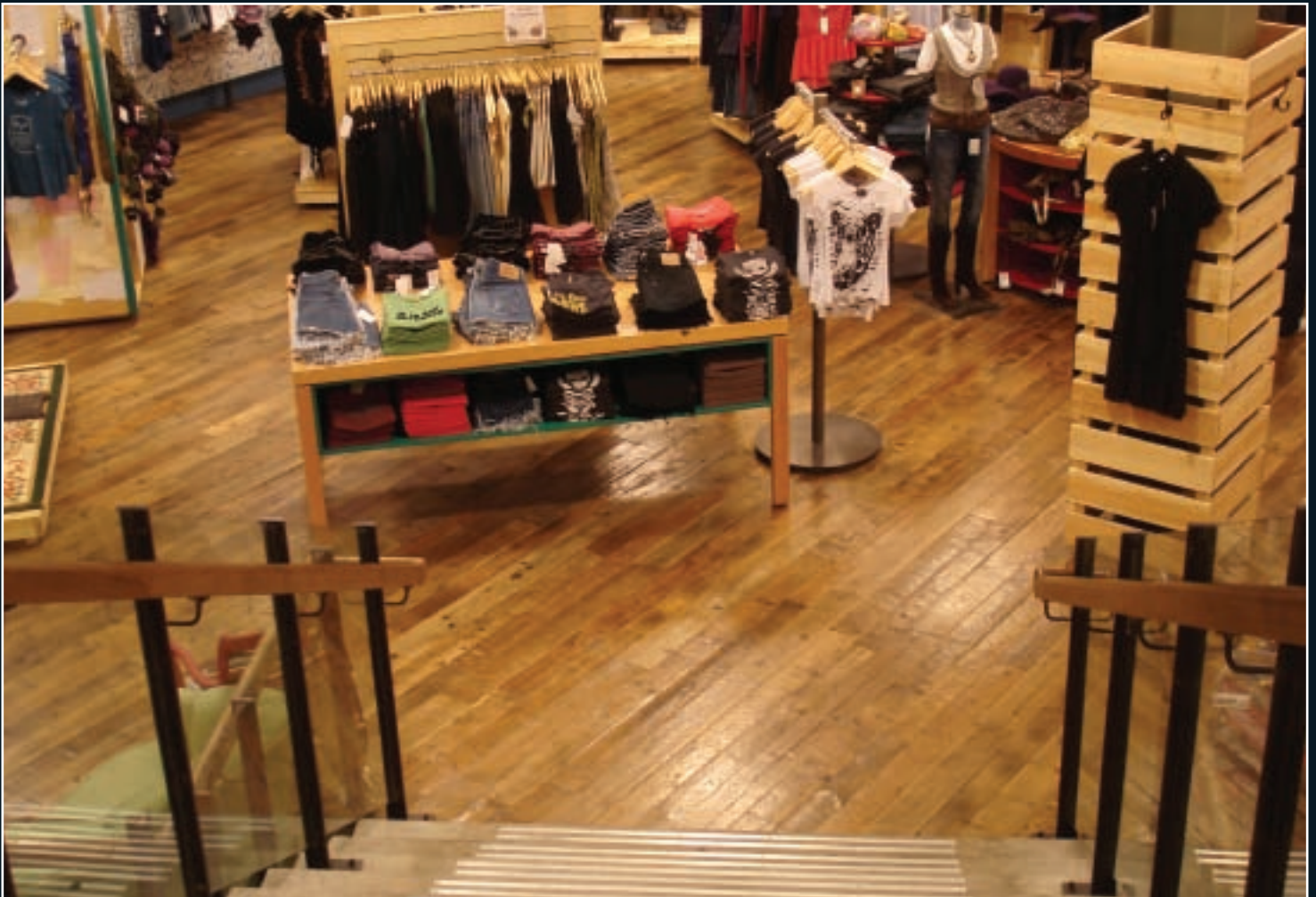
URBAN OUTFITTERS. Chesley Square Texture. Supplied "In the White", but filled and DA Sanded. Finished on site. Alpha 1 – Satin.
