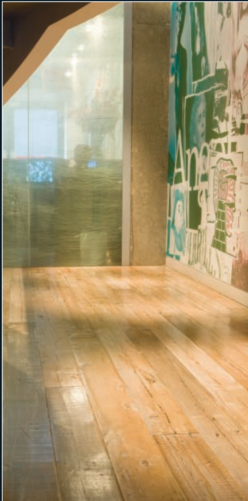
Sony HQ Entrance and Communal areas. Chester Square Texture – with deliberate “Country” or “Rustic” effect. Soap One. UV Lacquer – Gloss.
